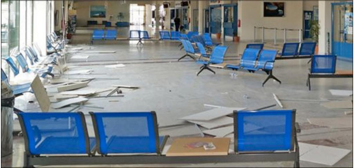
**Figure 2-9.** Suspended Ceiling Damage at Lemnos Airport (After Liz Fields (/contributor/liz-fields))
