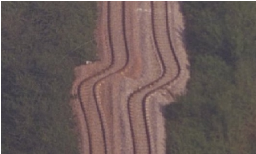
Figure 27. Bucking of the railroad track near Sapance in Kocaeli Earthquake
