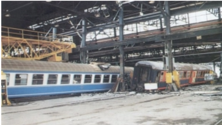
Figure 21. Damage at TUVESAS rail car factory (steel building) in Adapazari
