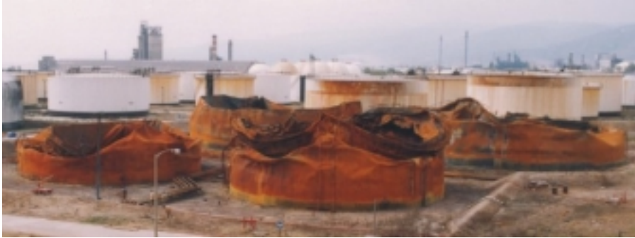
Figure 32. Post-earthquake fire damaged tanks in Tupras petrochemical complex
