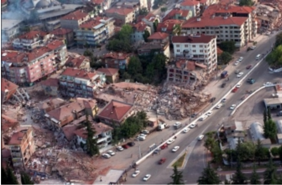
Figure 16. A general view of building damage in Golcuk
