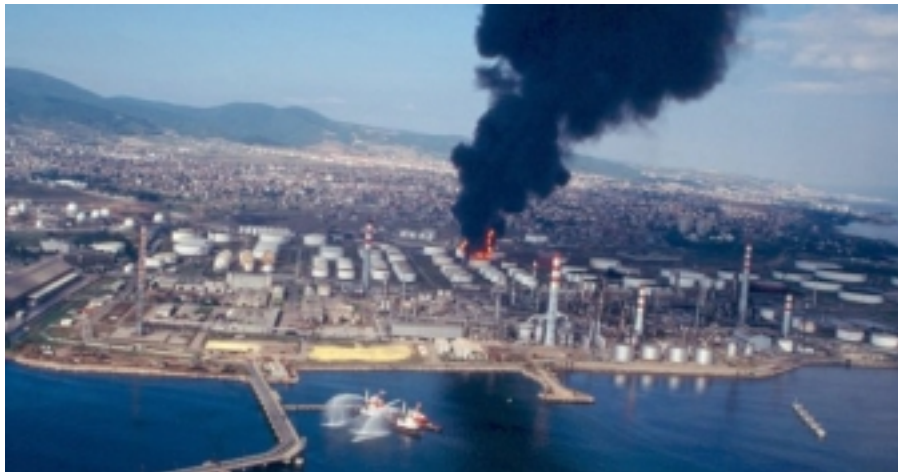
Figure31 A helicopter view of the fire in Tupras petrochemical complex.
