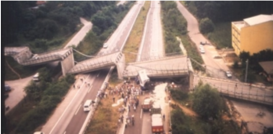
Figure 24. Collapse of the Arifiye overpass on TEM Highway in Kocaeli Earthquake.
