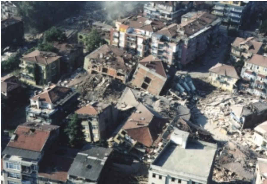
Figure 17. A general view of building damage in Duzce
