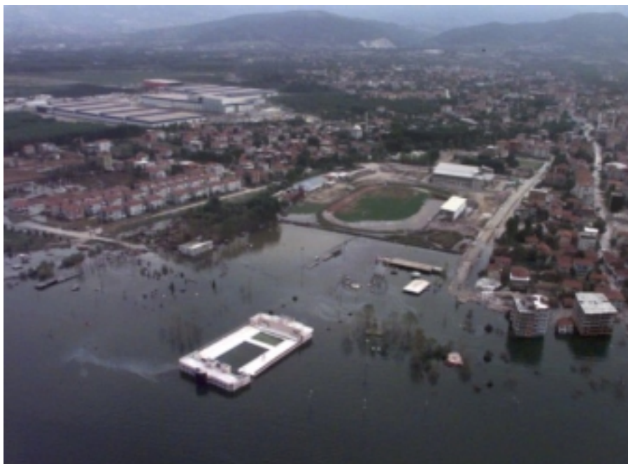
Figure 15. Subsidence at Golcuk along the southern shore of the Izmit Bay
