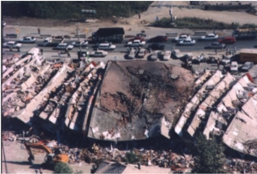
Figure 18. A “pancake” type collapse in Kocaeli Earthquake
