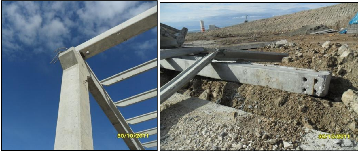
Figure 16. Failure of precast beams due to weak connection and lack of steel bondage
