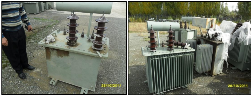
Figure 20. Damage to brittle bushings due to fall of building elements onto the interconnecting cables
