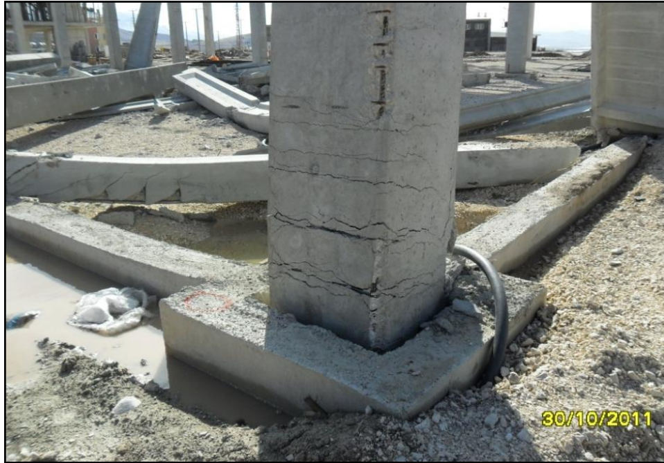
Figure 18. Cantilever column bending cracks at the base
