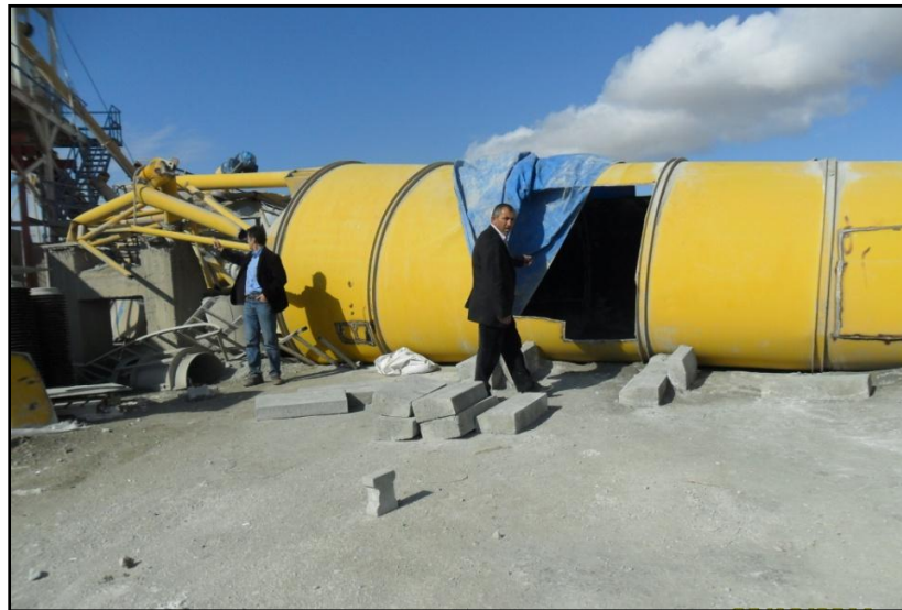
Figure 7. Collapsed cement silo in the Van Industrial Zone
