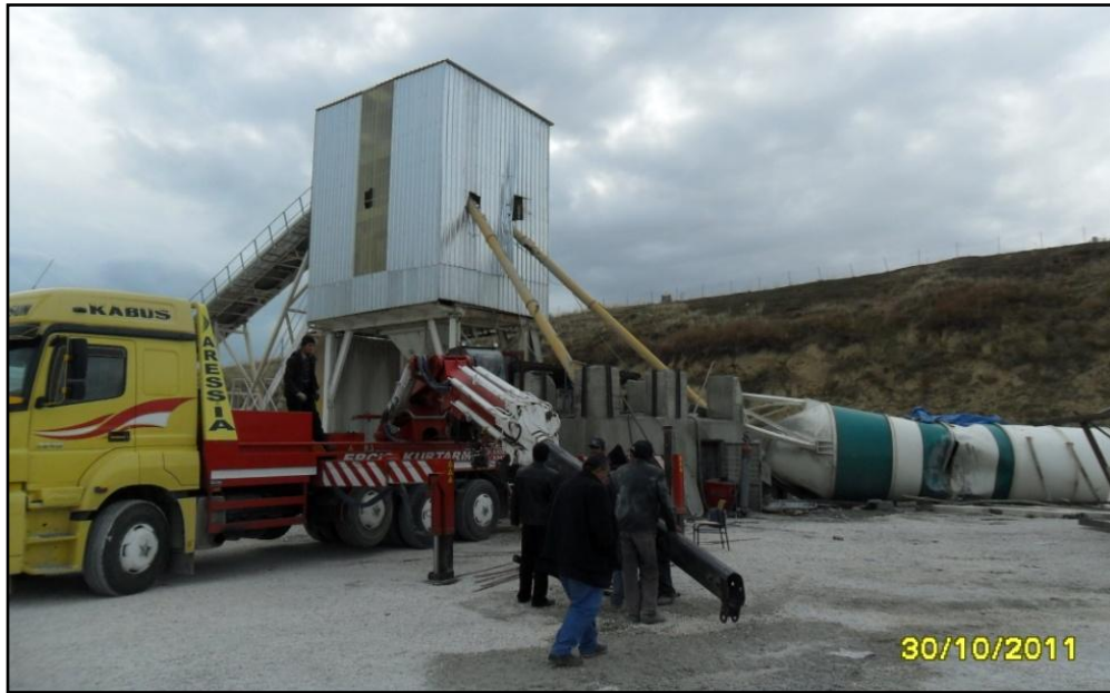
Figure 9. Collapsed silo on the Ercis-Patnos highway due to failure of the supporting concrete
