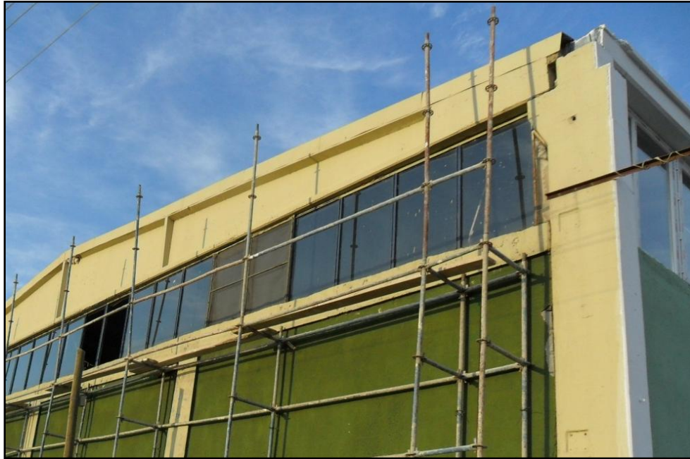
Figure 14. Joint separation in prefabricated structures
