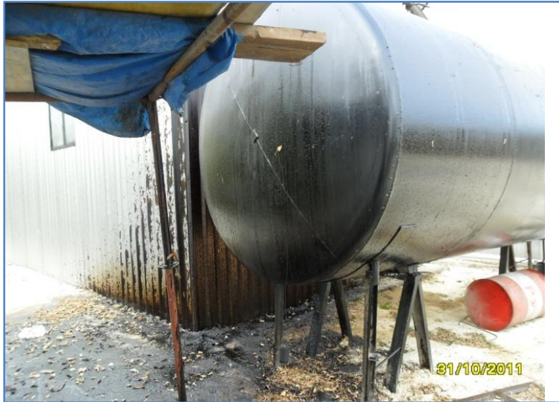
Figure 12. Overflow of liquid at elevated fuel oil tank (Ercis)
