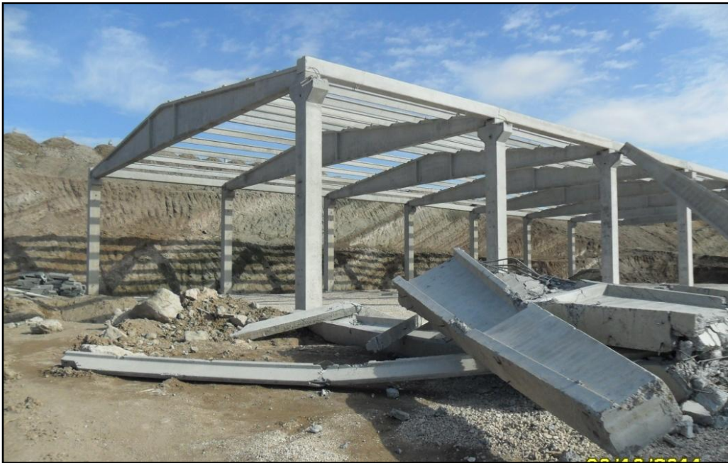
Figure 15. Collapsed prefabricated structure in Van Industrial zone (Facility 1)
