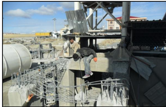
Figure 8. Damaged cement silo in Van Industrial Zone due to concrete crashing
