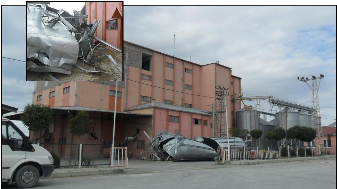
Figure 10. Collapse of the elevated wheat silos (Facility 1) due to inadequate dimensioning, Van
